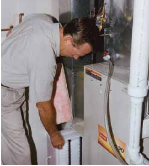
Checking a deep-pleated air cleaner.
