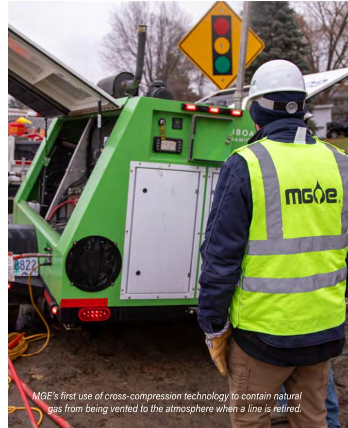
*MGE's first use of cross-compression technology to contain natural gas from being vented to the atmosphere when a line is retired.*
