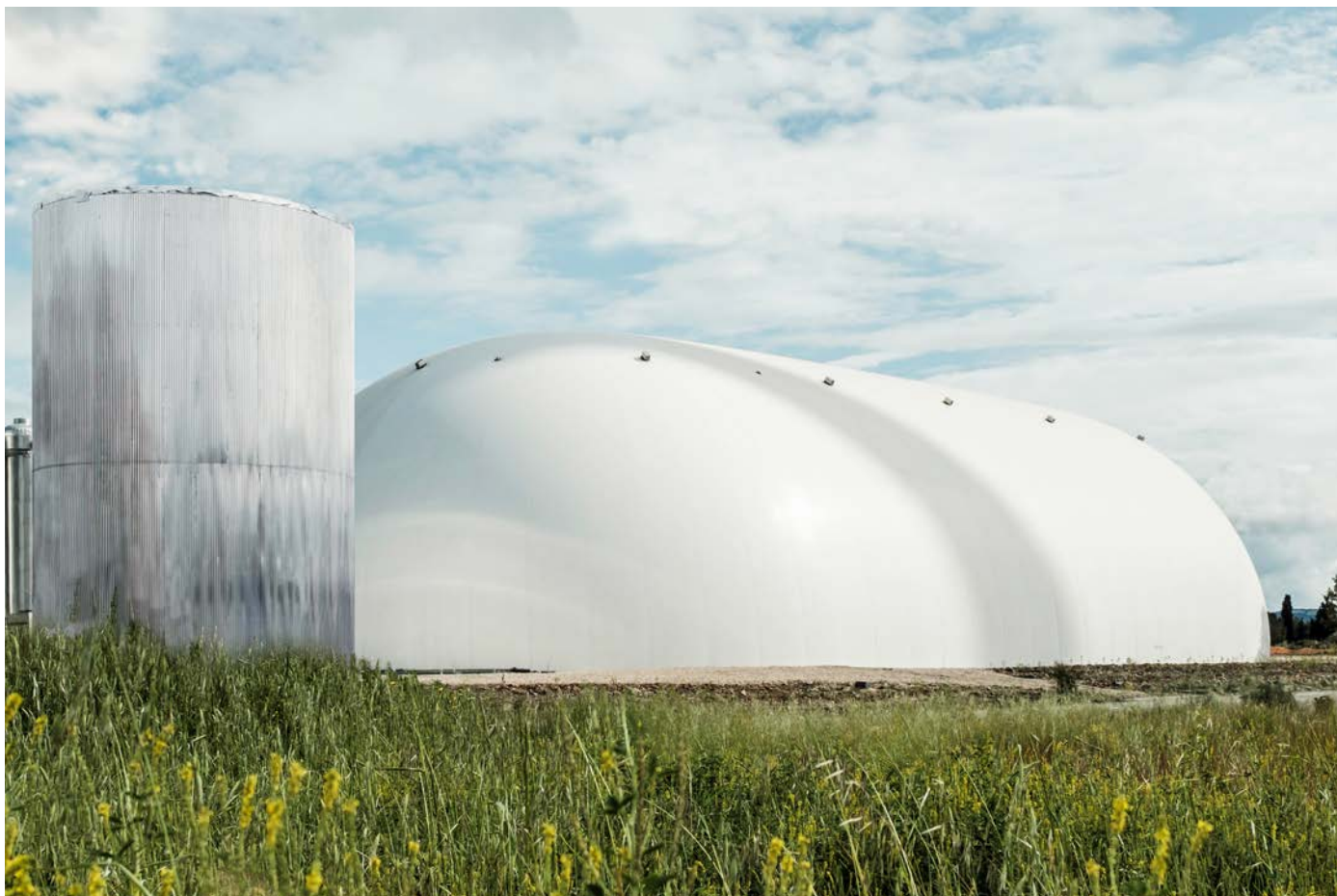
Courtesy: Energy Dome, Alliant Energy
