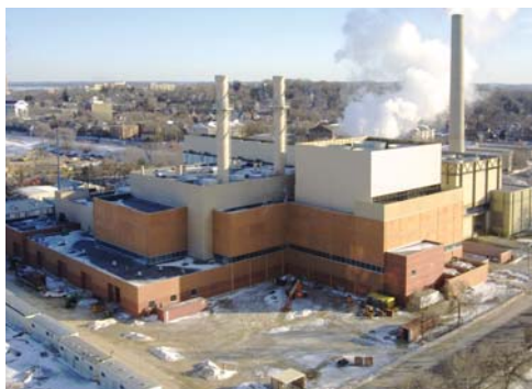
The new cogeneration facility will provide steam for heating and cooling UW campus buildings and serve as a vital new source of electricity for our growing area.
