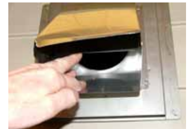
Vent termination with backdraft damper
