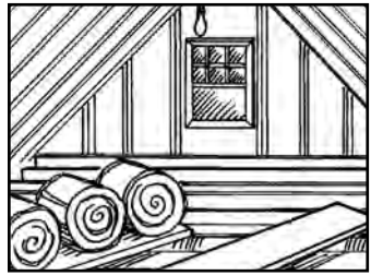
Figure 3 - Install temporary floor and lighting in the attic.
